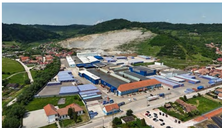
Leier ROM plant Sighisoara, County Mures
