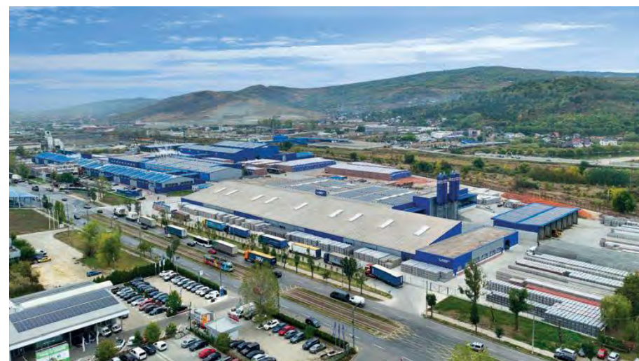
LEIER ROM Iasi Plant
